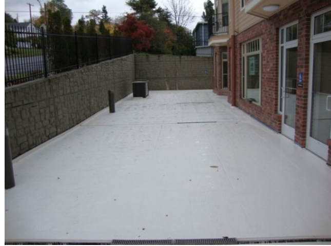
Ultra Flex Waterproofing System EP-990C Base, UFECO5000 Intermediate Coat, UF6800 Non Skid Traffic Coat
